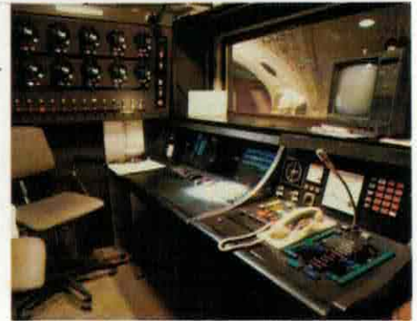
Strand Lighting in Vienna - installed by Ludwig Pani. Above: the Galaxy system at the Vienna State Opera (also in view, extreme left, is the Pani PEF-M remote control for motorised spotlights). Right (top): A Galaxy at the Theater in der Josefstadt. Right (lower): A Light Palette at the Volkstheater.
