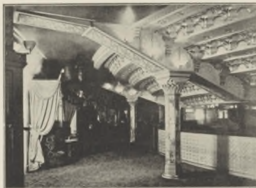
"ALHAMBRA" VARIETY THEATRE, LONDON. VIEW OF FENESTRATION.
