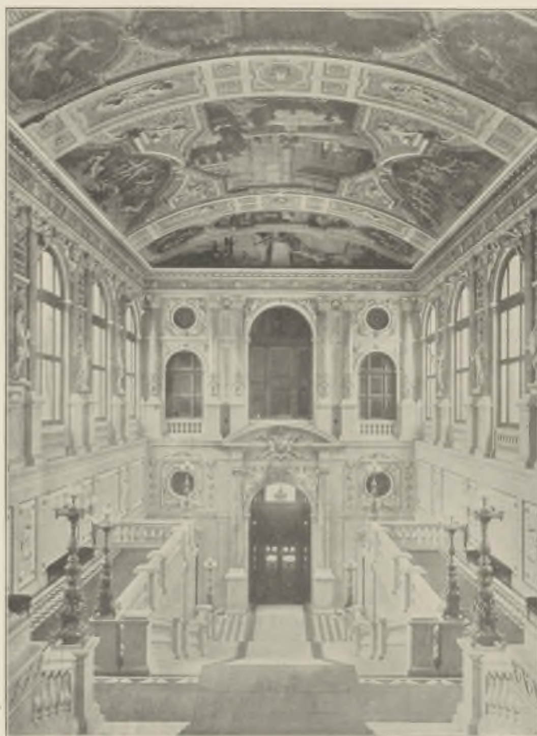
COURT THEATRE, VIENNA. VIEW TO ENTRANCE END OF GRAND STAIRCASE.
