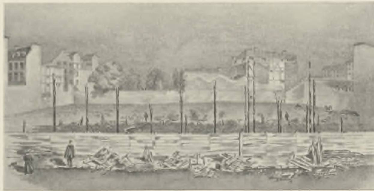
TEMPORARY THEATRE, PARIS (KNOWN AS CHARITY BAZAAR). Destroyed MAY 4, 1897. FIG. 2. GENERAL VIEW AFTER FIRE.
