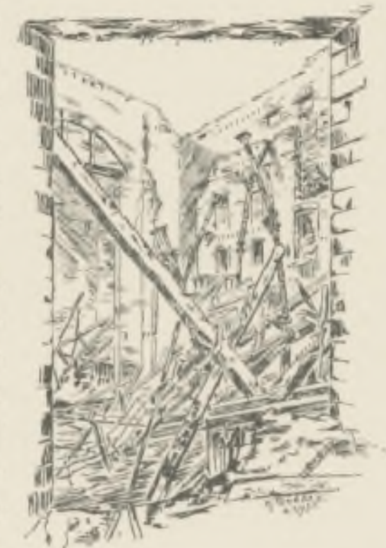
THEATRE "ROYAL," GLASGOW. Destroyed March 1, 1895. FIG. 17. VIEW OF AUDITORIUM AFTER FIRE.
