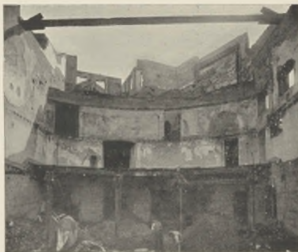
THE THEATRE, EXETER, Destroyed SEPTEMBER 5, 1887. FIG. 7. VIEW OF AUDITORIUM AFTER FIRE.
