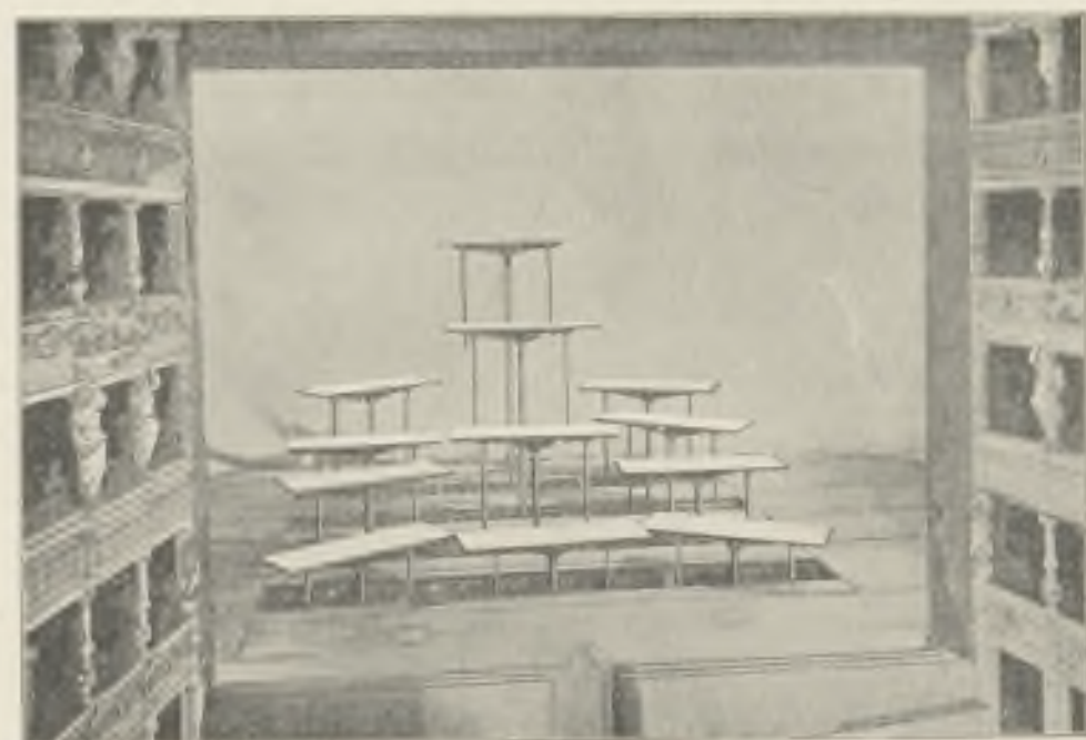
THE 'ASPHALEIA' SYSTEM: STAGE. FIG. 68. DIAGRAM SHOWING 'BRIDGES.'
