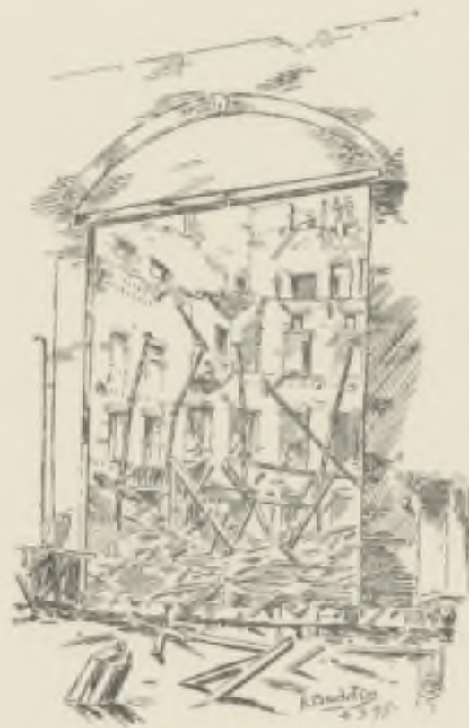
THEATRE "ROYAL," GLASGOW. Destroyed March 1, 1895. FIG. 16. VIEW OF AUDITORIUM AFTER FIRE.
