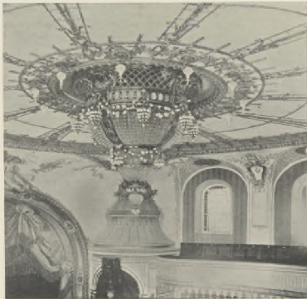
MUNICIPAL THEATRE, BROMBERG. AUDITORIUM. FIG. 451. VIEW OF 'HIDDEN SKYLIGHT.'
