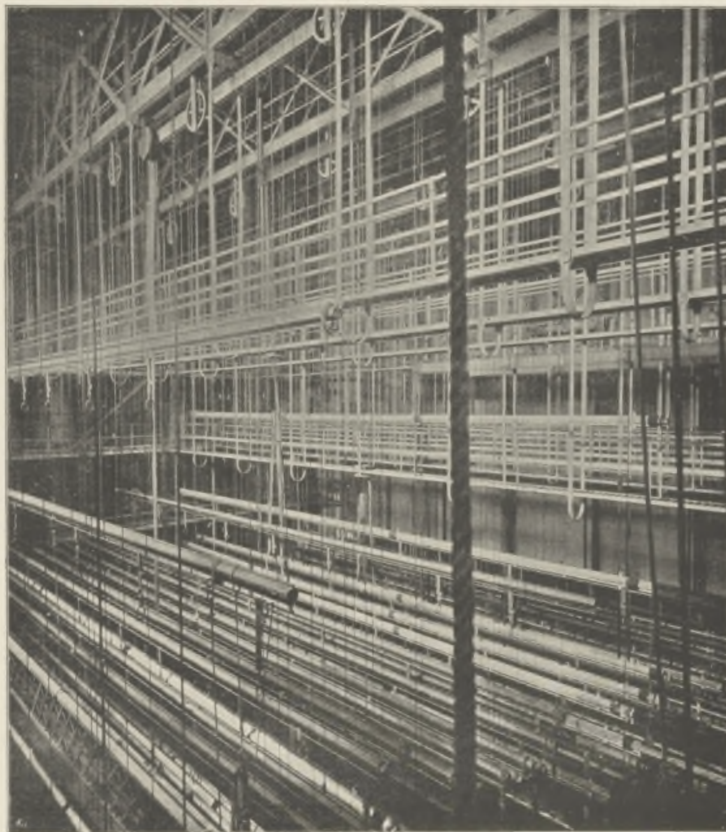
COURT THEATRE, VIENNA. STAGE. FIG. 84. VIEW OF 'UPPER MACHINERY'
