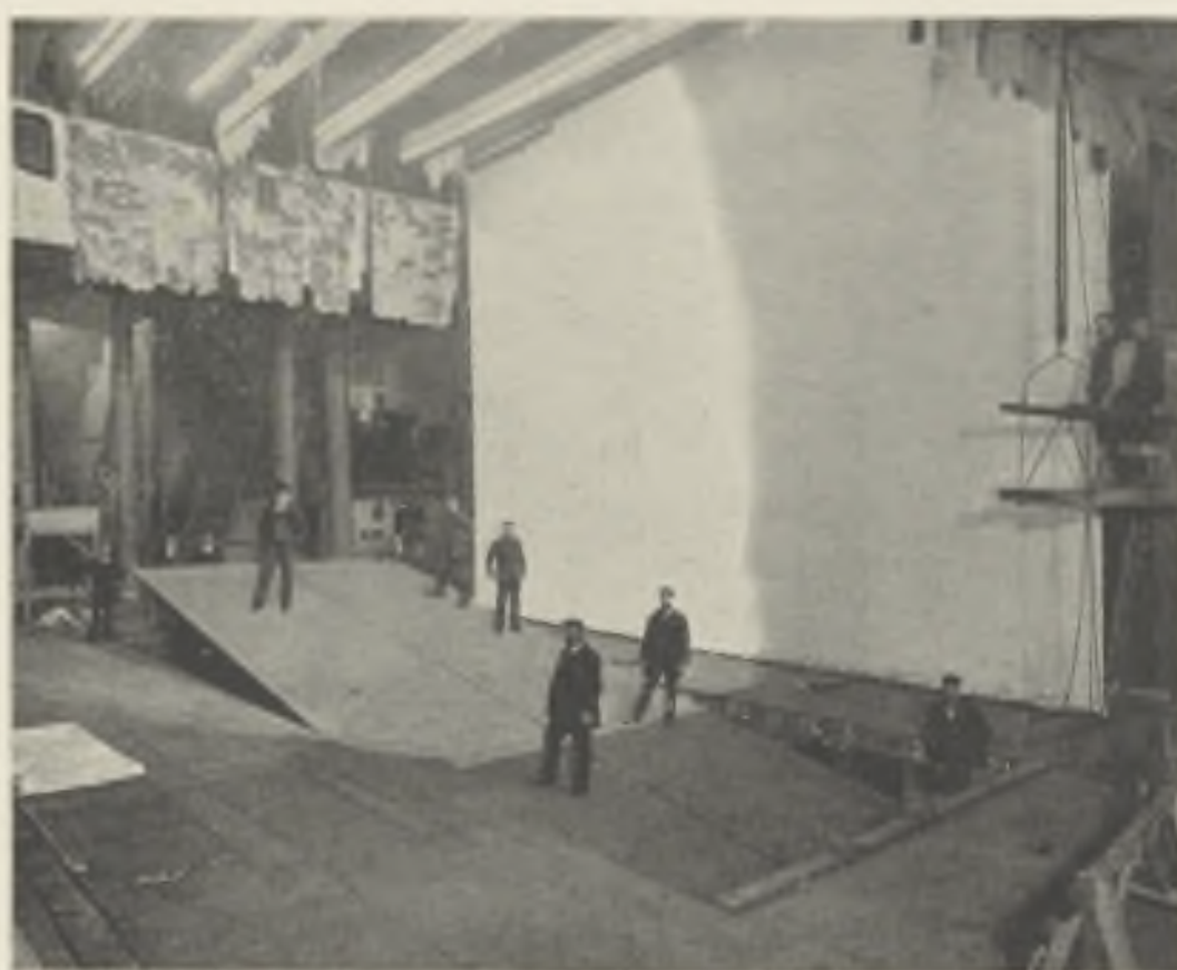
DRURY LANE THEATRE, LONDON. STAGE. FIG. 2. VIEW OF HYDRAULIC 'BRIGGS' IN SLOPING POSITION.
