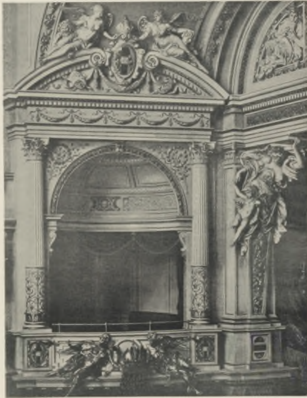
COURT THEATRE, VIENNA. FIG. 433. VIEW OF PROSCENIUM CORNER.
