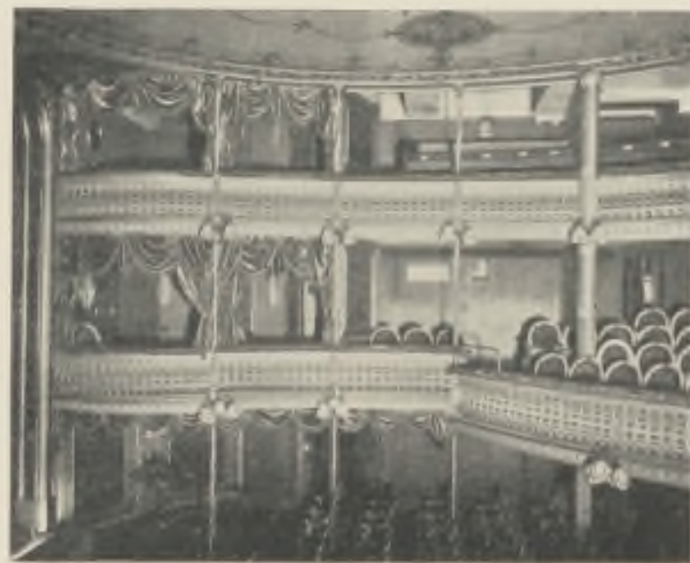
'CRITERION' THEATRE, LONDON. FIG. 254. VIEW OF AUDITORIUM.
