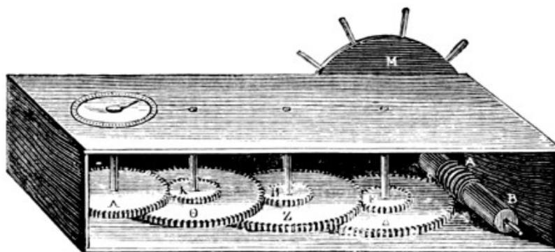
FIG. 2.—ODOMETER FOR VESSELS.
