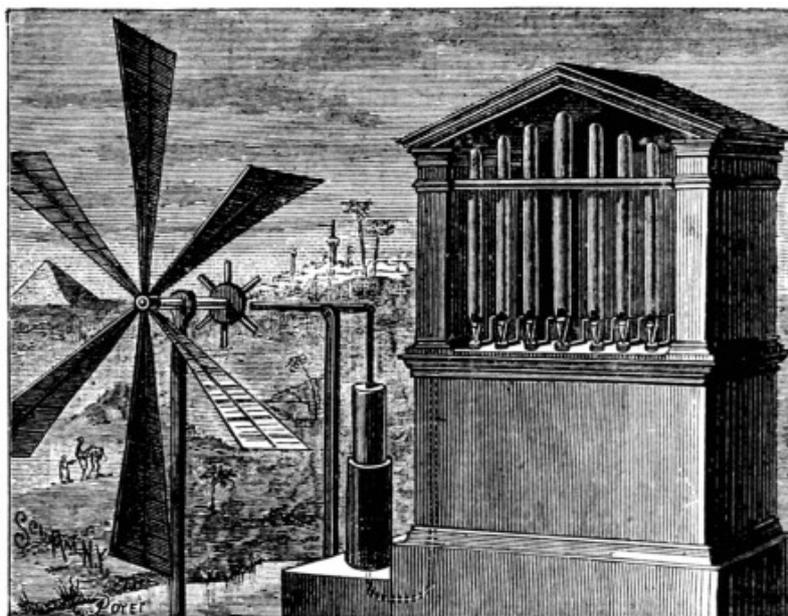
FIG. 4.—WINDMILL DRIVING THE BELLOWS OF AN ORGAN.
